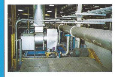
Duct work design and installation for transporting emissions from the process to thermal oxidizer and other control device.
